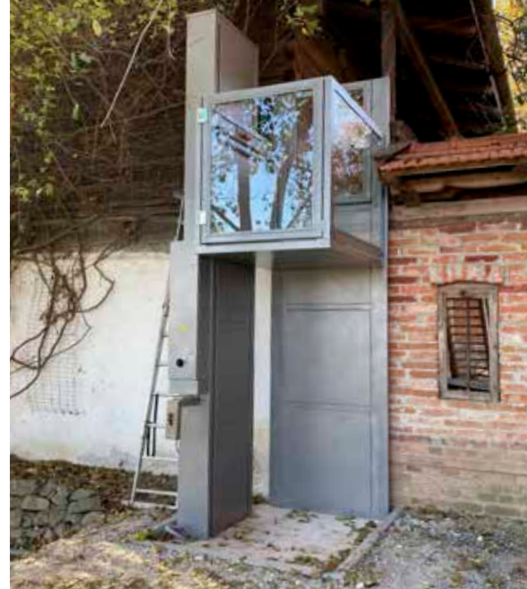
Safety glass at upper door, platform door and platform side walls
