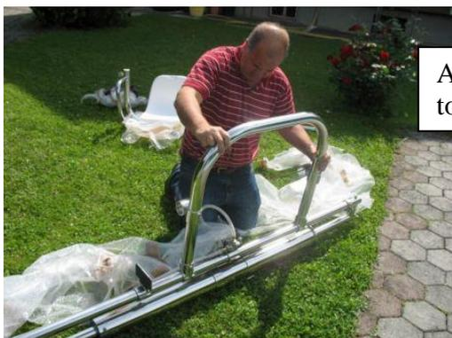
Applying the C-tube and screwing it together
