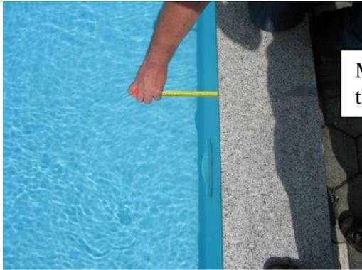
Measuring out the overhanging of the pool edge
