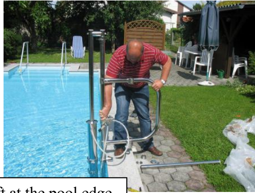
Placing the Poollift at the pool edge
