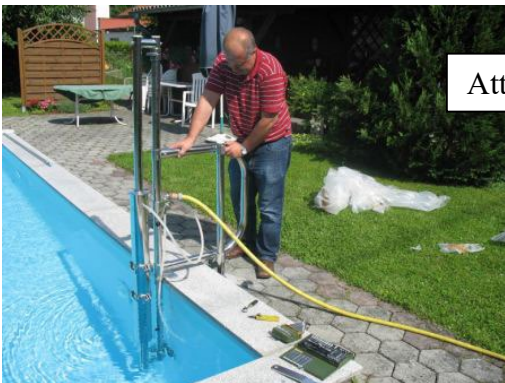
Implementing the additional pillar and screwing it to the panel using the union nut
