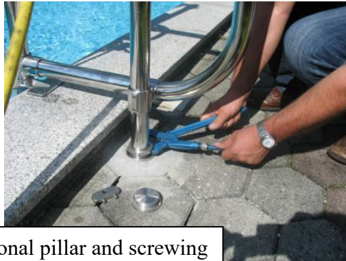
Placing the Poollift at the pool edge
