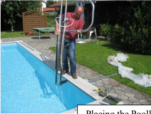
Placing the Poollift at the pool edge
