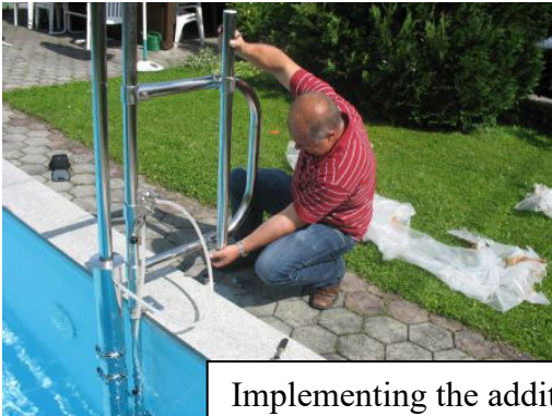
Placing the Poollift at the pool edge
